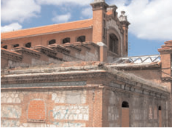
Vista exterior alzado principal
