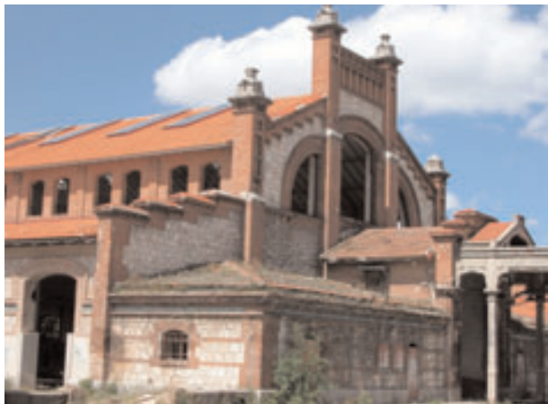
Vista exterior alzado principal
