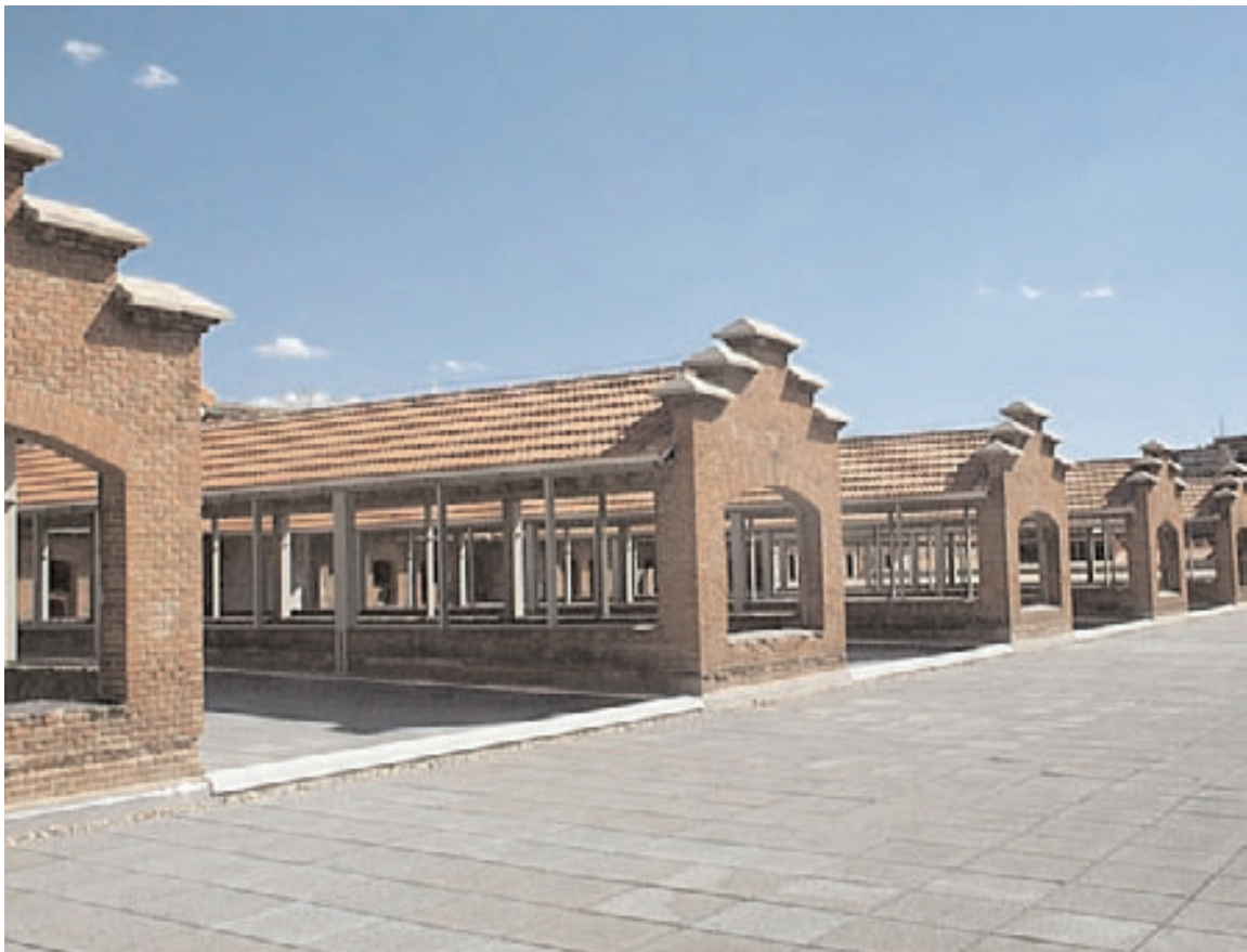
Vista exterior lucernarios
